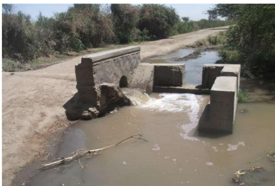
Flow division structure with missing control gates at Meki Ziway irrigation scheme
